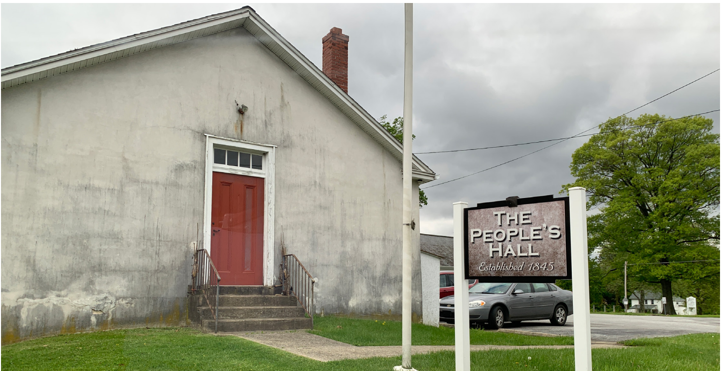
The People's Hall, built in 1845 as a meeting place for the East Fallowfield Anti-Slavery Society
