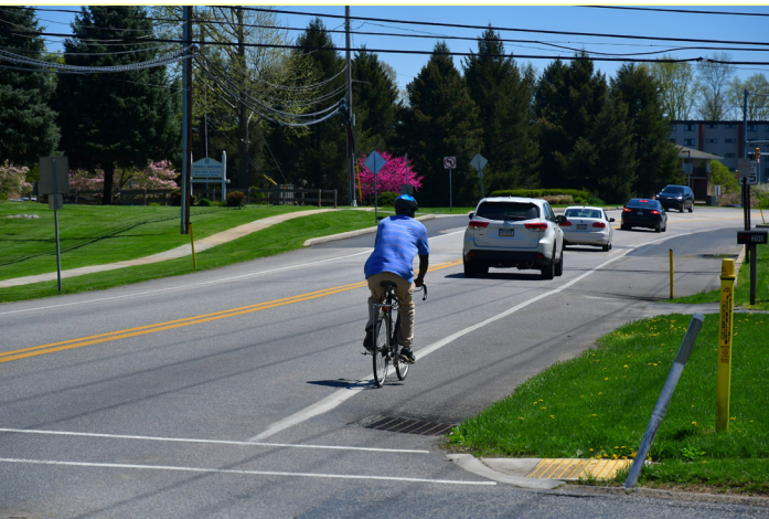
Above: Examples of shoulder improvements
