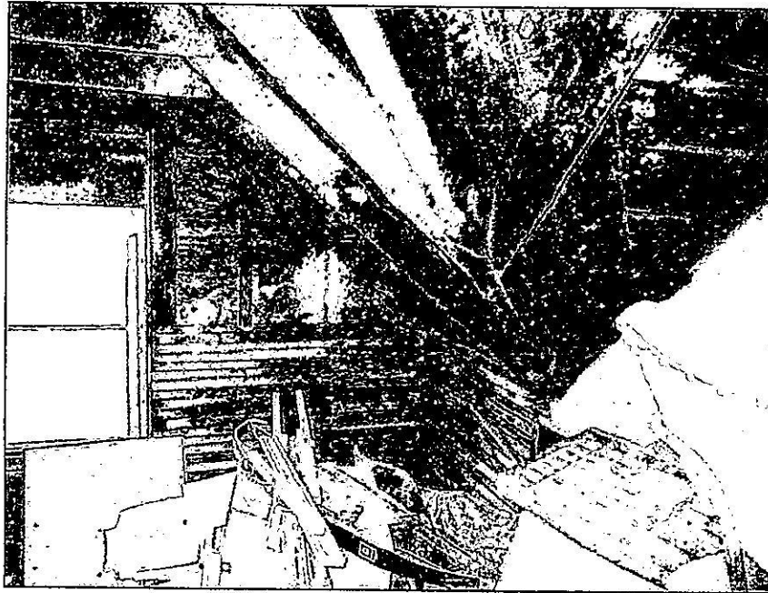
Photo 20: SDA observe common nail roof framing in the 3 rd floor attic area.
