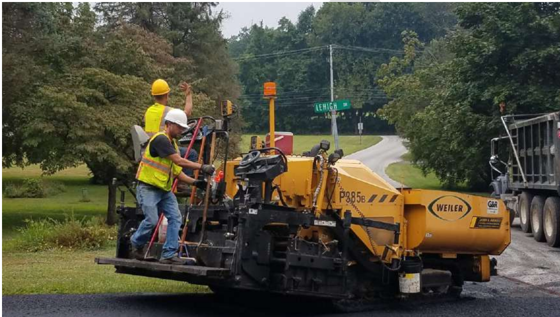
Township road paving project
